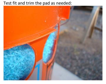
When the pad fits correctly, silicone or hand stitch the seam with needle and thread. This will give you a cylinder ~13 inches tall:
